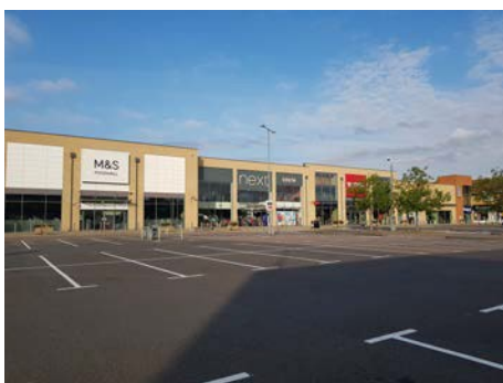
New units in Chequers Court, Huntingdon
